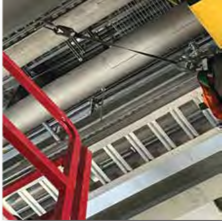
Strut Anchor in place on a job site.
